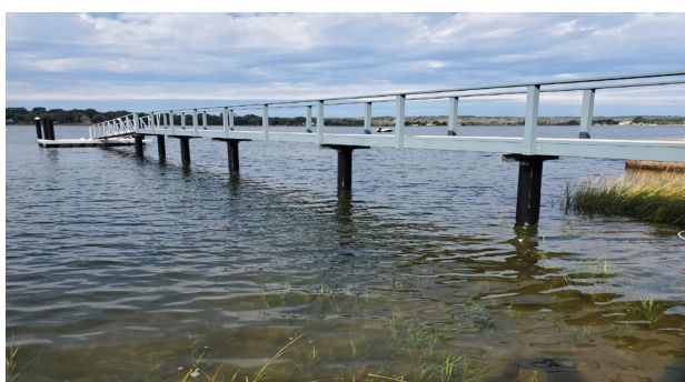
Pearson Pilings All Composite Dock, Berkley, MA
