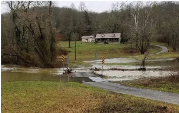
Photo of Morgan County Bridge which is being replaced
